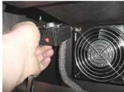
A 3/16 bolt already welded in the interior allows to fix the thermodisc box. Two holes on the left side of the fireplace are provided to take out the wire (a connector is necessary).
