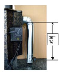
➤ Position the 90 degrees elbow and the 6 inches diameter coated sheet pipe (or black steel). Fix the 90 degrees elbow only with screws of less than ½" of length because it could affect the good operation of the anti-repression valve.
