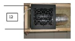
Screw the basement ceiling grid with 6 screws of 1 <sup>1</sup>/<sub>2</sub>". The necessary space between the joists must be of 12 inches centre in centre. Be sure that the box does not touch the joists in order to avoid noises.
