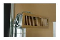
➤ Install the fan conducts without any clearance from the ceiling. At each conduct extremity, install a floor grid.
