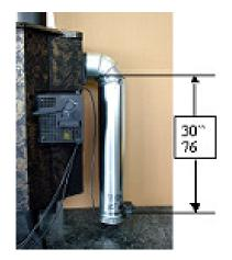
Position the 90 degrees elbow and the 6 inches diameter coated sheet pipe (or black steel). Fix the 90 degrees elbow only with screws of less than ½" of length because it could affect the good operation of the anti-repression valve.
