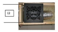
Screw the basement ceiling grid with 6 screws of 1 ½". The necessary space between the joists must be of 12 inches centre in centre. Be sure that the box does not touch the joists in order to avoid noises.
