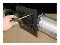
Screw the fan grid (GV460) by using 5 bolts (1" X ¼") with locks.
