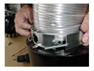
Install the retaining collar with 2 bolts and nuts (1/4 " X 2 ") and then tighten the end on the simple pipe.
