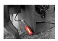
Pass the fan power supply wire into the connector and let it exceed of 6 inches in the protection box.
