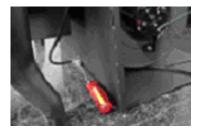
➤ Pass the fan power supply wire into the connector and let it exceed of 6 inches in the protection box.
