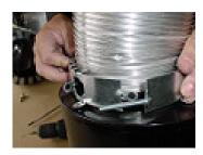
➤ Install the retaining collar with 2 bolts and nuts (1/4 " X 2 ") and then tighten the end on the simple pipe.
